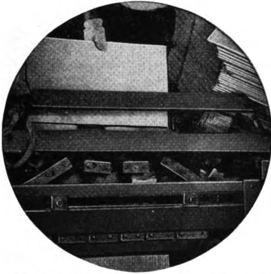
Trimming and nail-punching asbestos-cement shingles.
